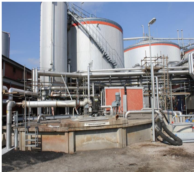
Fig. 7. Wet fermentation of separated communal waste in Linköping – Sweden
