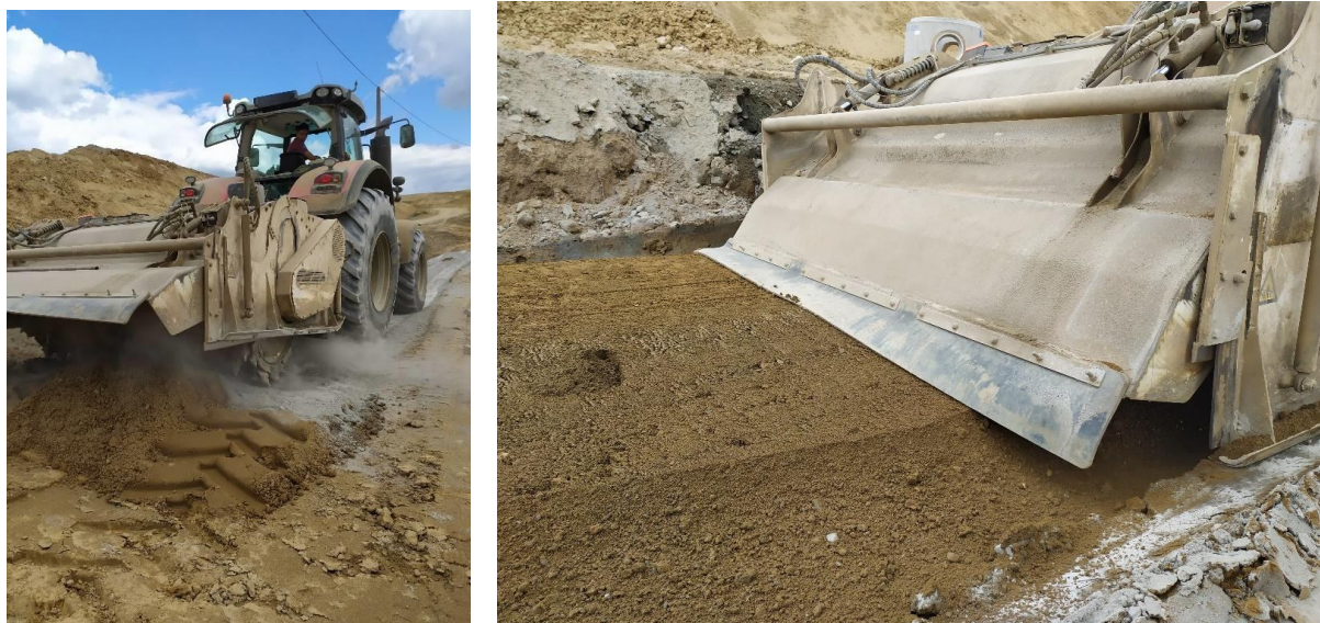
Fig. 20. The soil and binding material mixing and road finishing.
