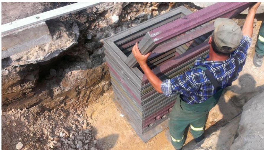
Fig. 19. Well construction elements from plastic waste
